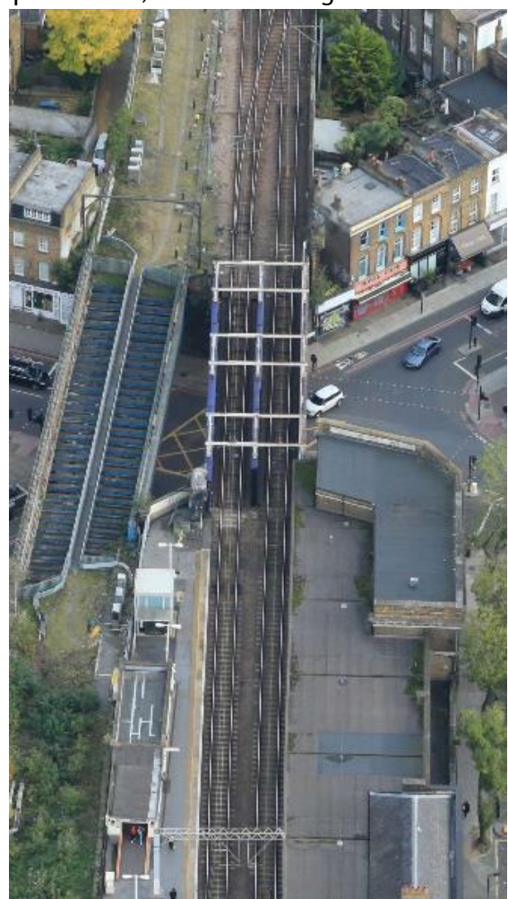
Aerial view of Camden Road Station looking to the East, with out of use track bed on the left. Source: NR RouteView
