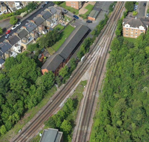
Aerial view of Nunhead Junction, looking west towards Nunhead station. The route towards Lewisham is to the bottom right. Source: NR Routeview
