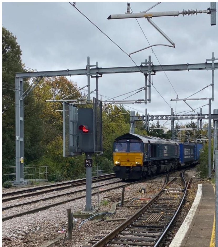
Source: Network Rail
