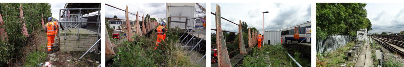
Existing lineside equipment. Source: '148508-ARP-SKT-EOI-000002 Existing Lineside Equipment Plan View', Arup for Network Rail (17/04/16)
