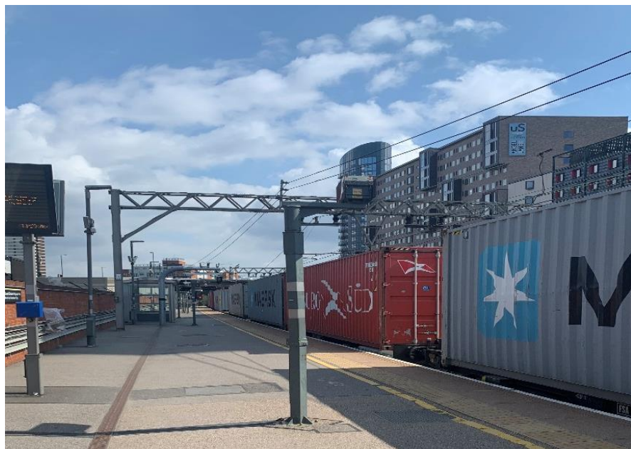
Platform 10a at Stratford station. Source: Network Rail
