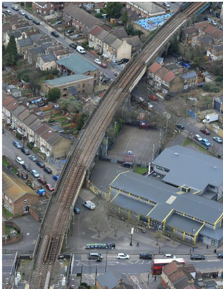
The GOB, looking west from Wanstead Park station, on viaduct and succession of underline bridges. Source: NR Routeview
