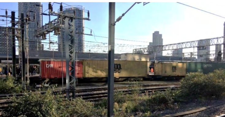
Source: Network Rail
