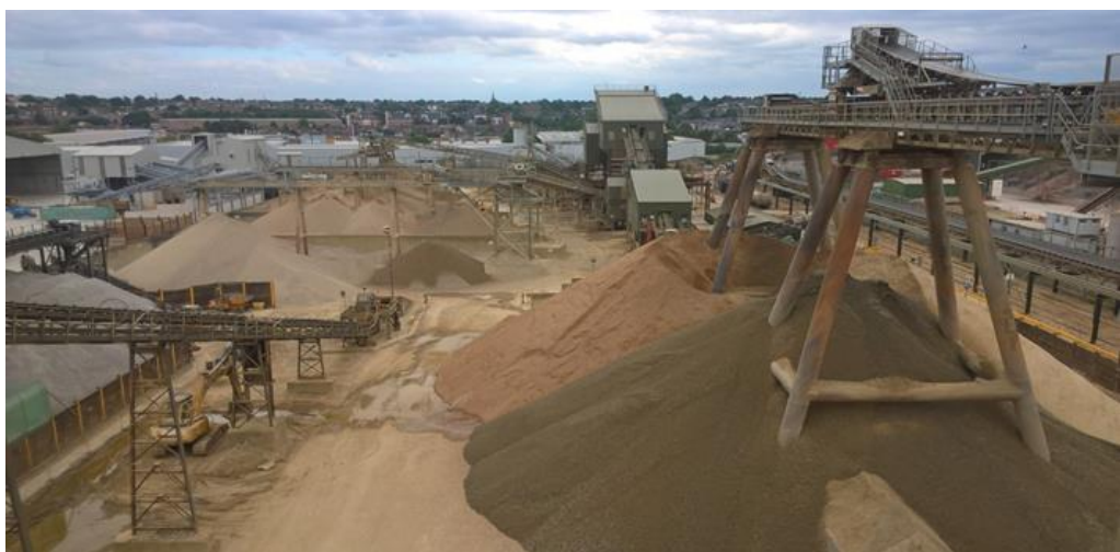
Stockpiles and hopper facilities for primary and secondary screening, at the Angerstein Wharf terminal. Source: Network Rail
