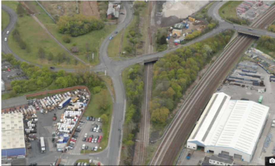
Siding connection into site off DSN line and under Metz Bridge. Siding will stay in SSFS boundary.
