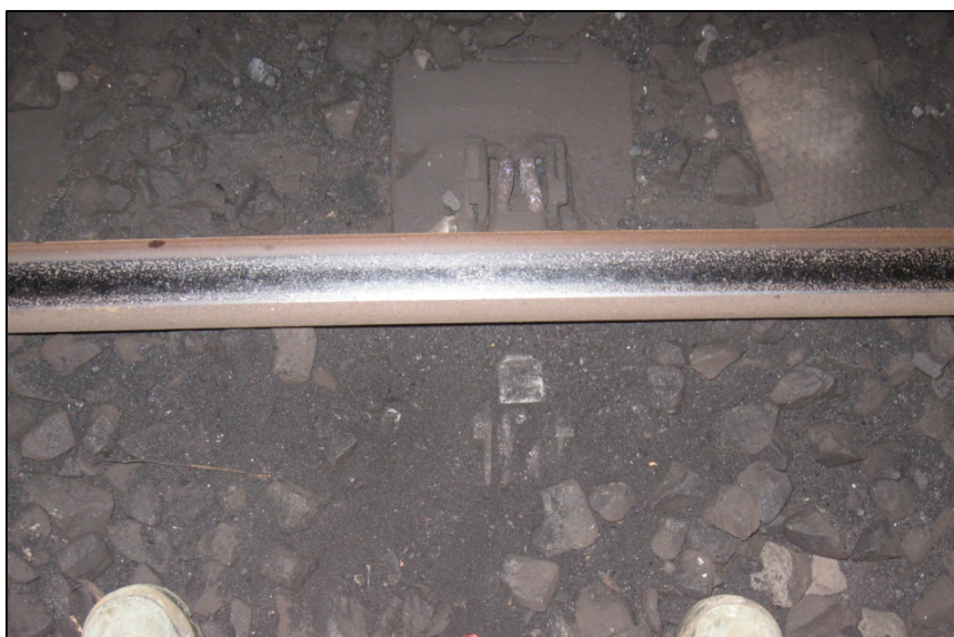
Fig. 6 Plain line in Severn Tunnel
