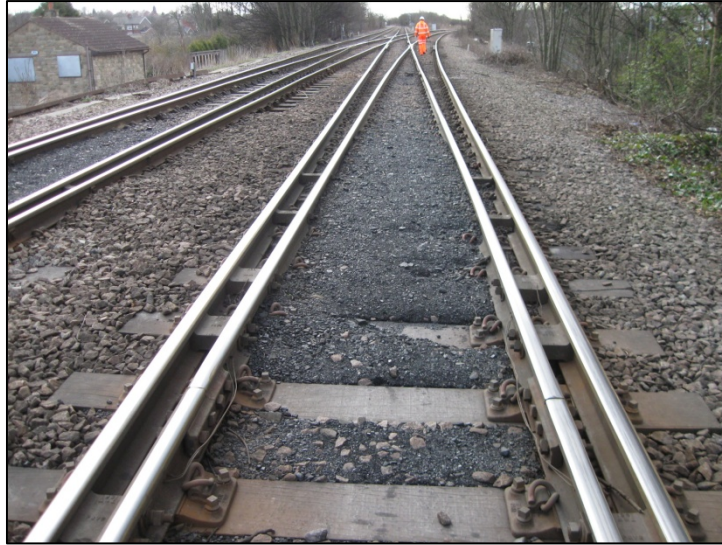
Fig. 4 Ferrybridge North Junction. Empty trains leaving Ferrybridge Power Station
