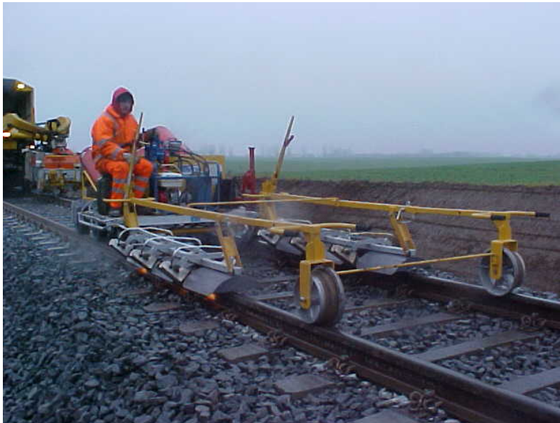
Picture: Rail heater trolley in action
