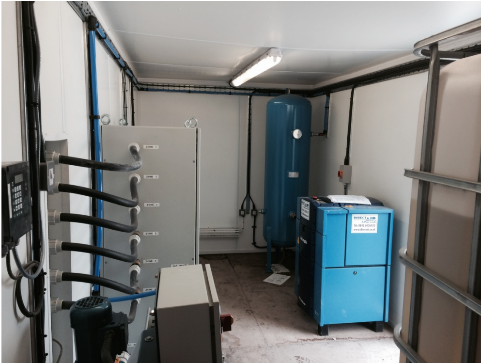
Photo 2 Internal view 2 of Modified Shipping Container
