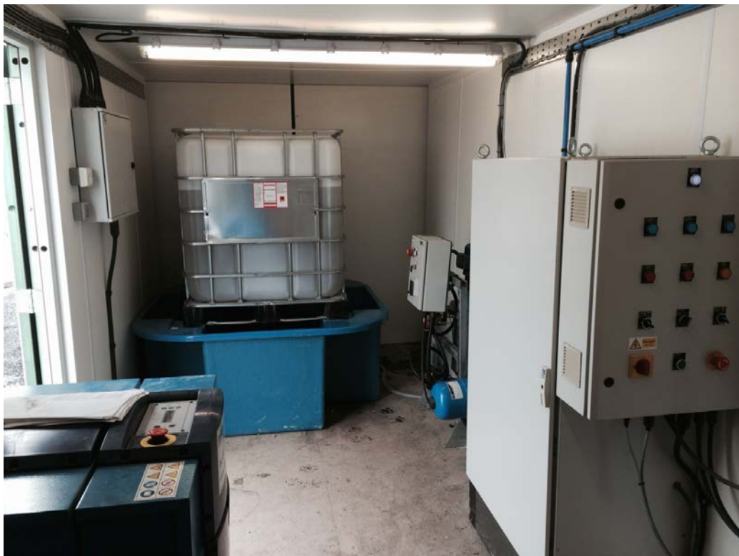
Photo 1 Internal view of Modified Shipping Container
