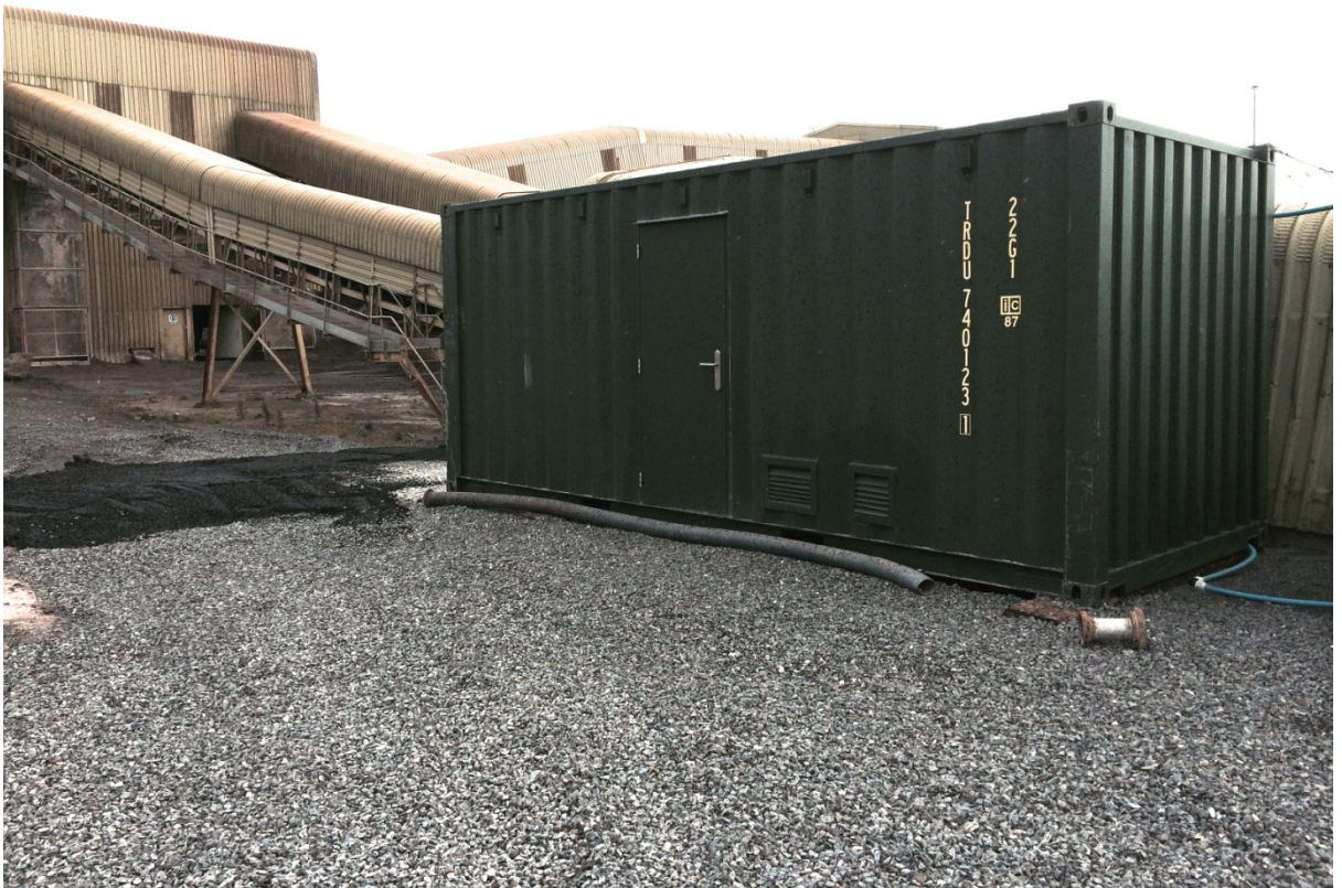
Photo 3 External view of installed (Bardon Hill) Modified Shipping Container
