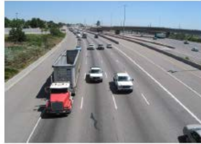
Level of Service B
